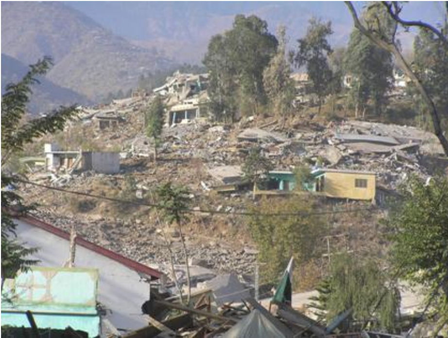
Figure 2: Collapsed and heavily damaged masonry residential units on a hill northwest of Balakot city centre
