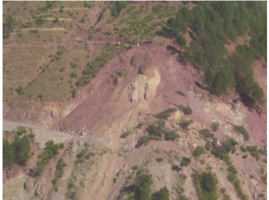
Figure 4: Landslide blocking the road to Balakot from the north (Photo: US Army)
