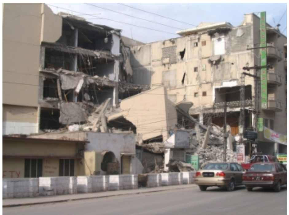
Figure 3: Collapsed part of a reinforced concrete hotel structure in Muzaffarabad city centre
